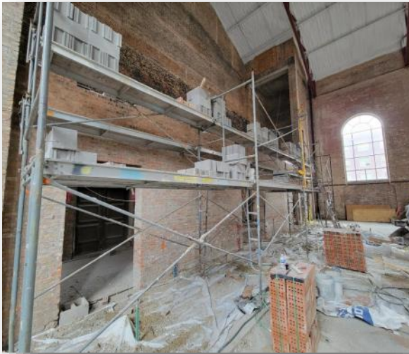
BUILDING UP THE VESTIBULE WALL FOR THE CHOIR LOFT FOUNDATION
