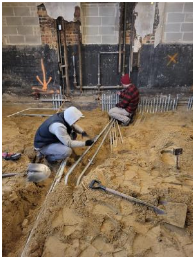
Electricians continuing Installation in basement
