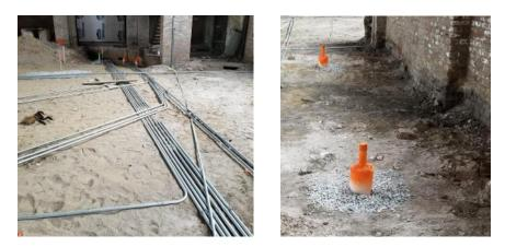
Conduit was run into the future basement, which was excavated to provide room for the future restrooms and infrastructure rooms. Access was cut under the sanctuary floor for plumbing and heating ducts. The drains for the "sacraria" or "blessed sink" were put into the nave, providing a direct access back to the earth for the water used for the washing of the hands during Mass at each of the many future side altars in the church.
