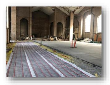
RADIANT HEAT TUBING HAS BEEN INSTALLED & LAID FLOOR SLAB HAS BEEN COMPLETED IN THE NAVE & NARTHEX INSTALLING WATER & ELECTRICAL INTO THE BUILDING
