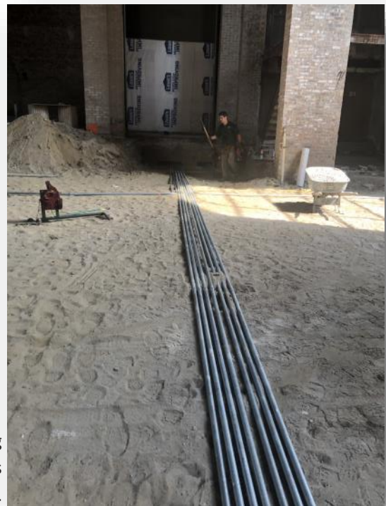
Electrical conduit being installed in the church this past week.
