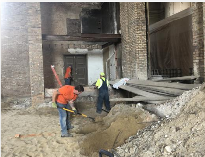
Plumbers working to install drainage system this past week.
