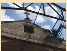
For the roofing diaphragm, most steel purlins are installed, while half of sag rods are installed. This week masonry work was done to repair the east pediment wall (photo) 70 feet up so that the purlins can be installed there early next week.
